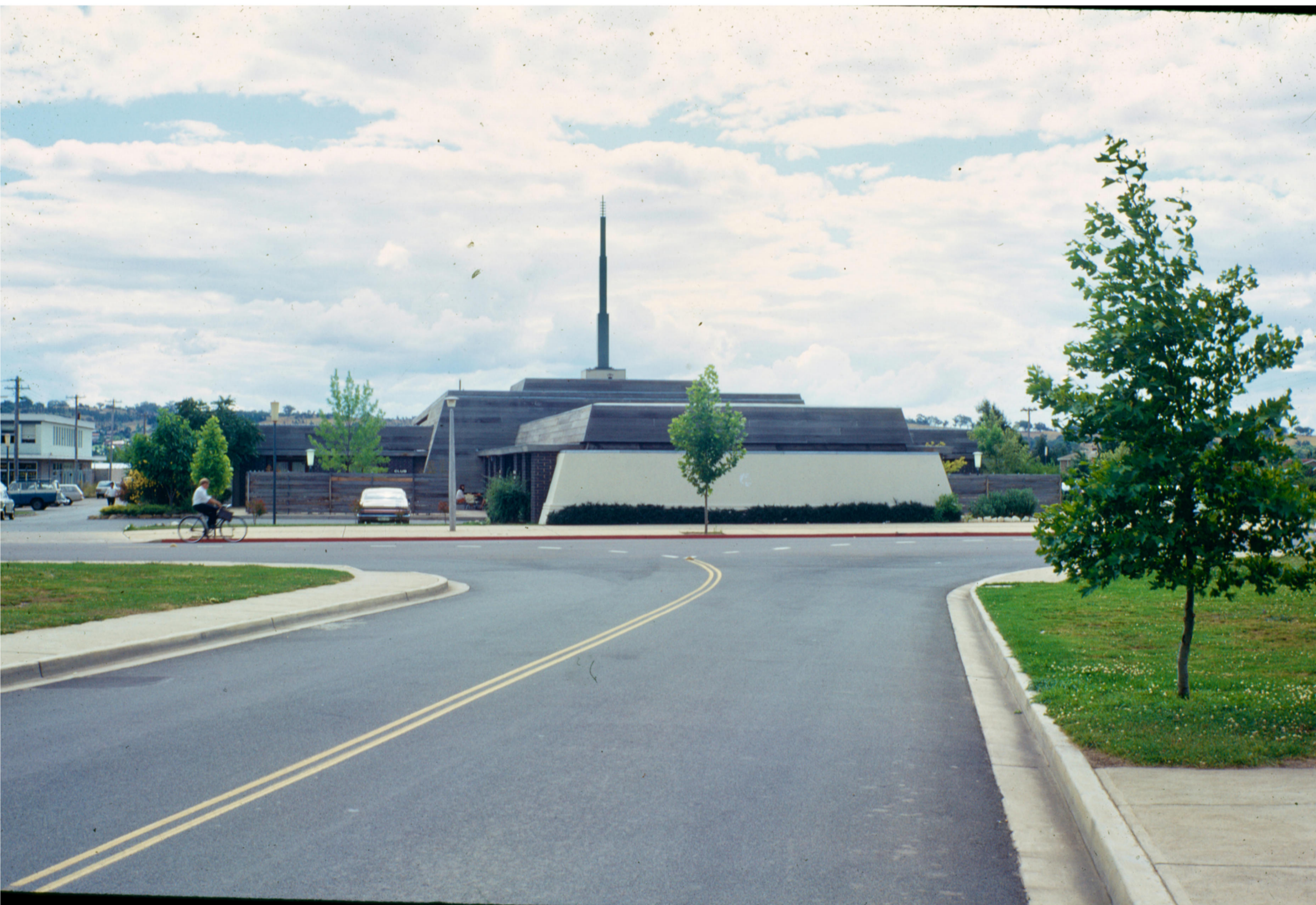
1966 Hotel Dickson by Peter Muller ( State Library of Victoria, photo by Peter Wille )
